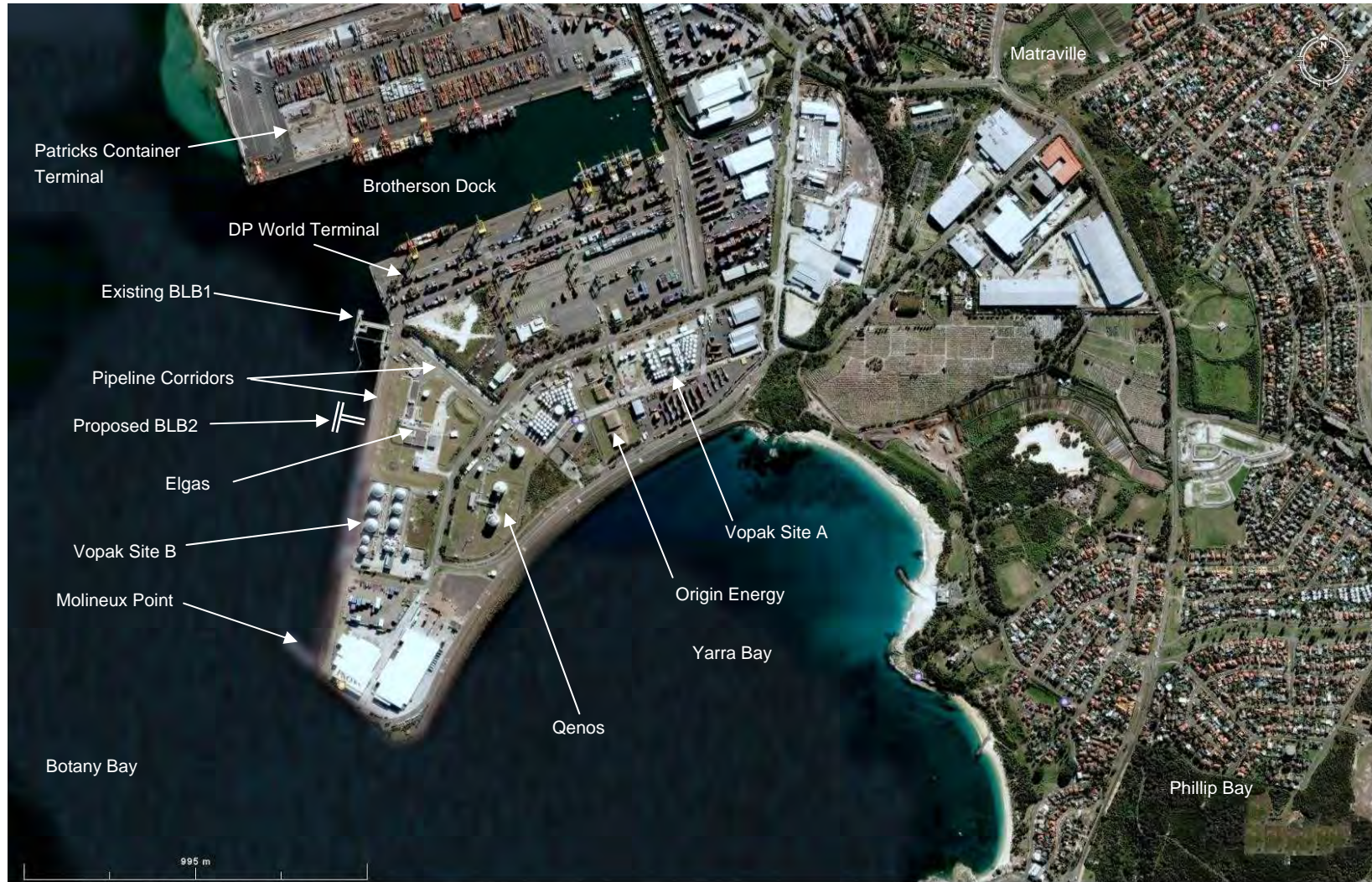
Figure 3-2 Aerial photograph of Port Botany showing BLB2 and surrounding land uses
