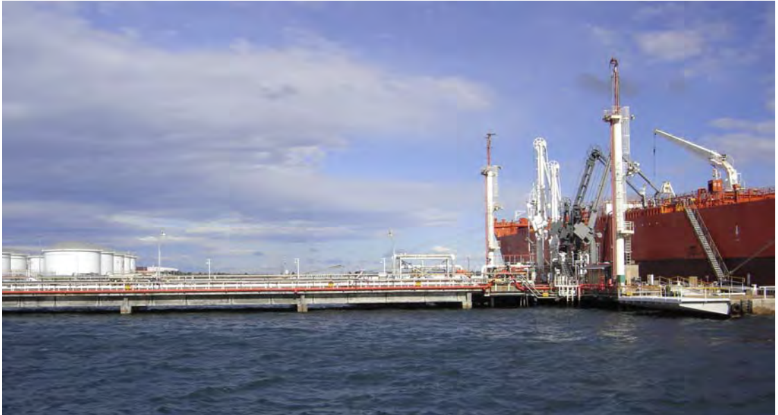
■ Figure 4-4 Existing BLB1 bulk liquids berth
