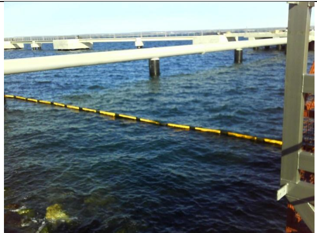
Photo 10 Silt curtain floating above surface with no gaps. (adjustments made by diver on anchoring)
