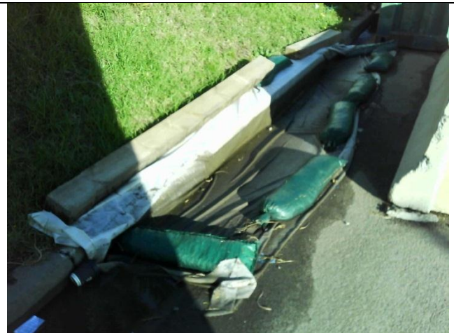
Photo 2 Drain well protected from sediment ingress adjacent to storage container
