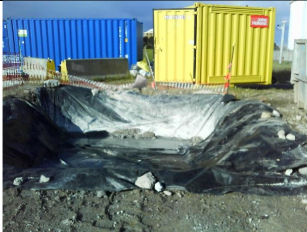
Photo 13 Concrete washout pit
