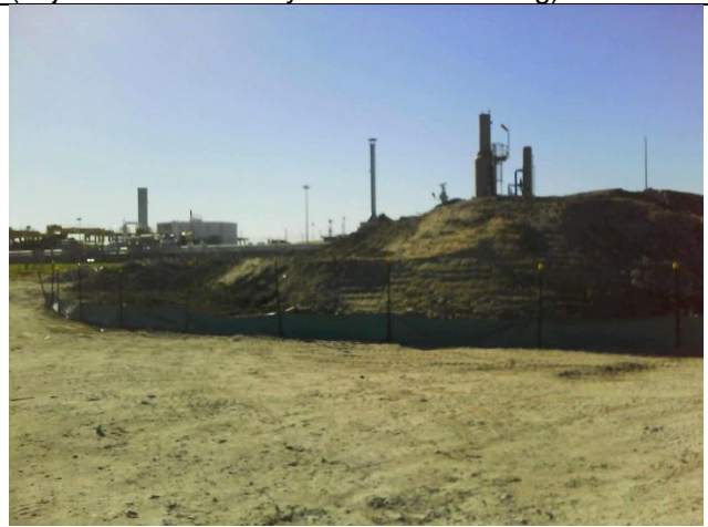
Photo 12 Sediment fence installed at foot of large stockpile. Stockpile battered.
