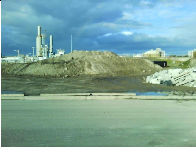
Photo 11 Main stockpile area – no downstream sediment controls
