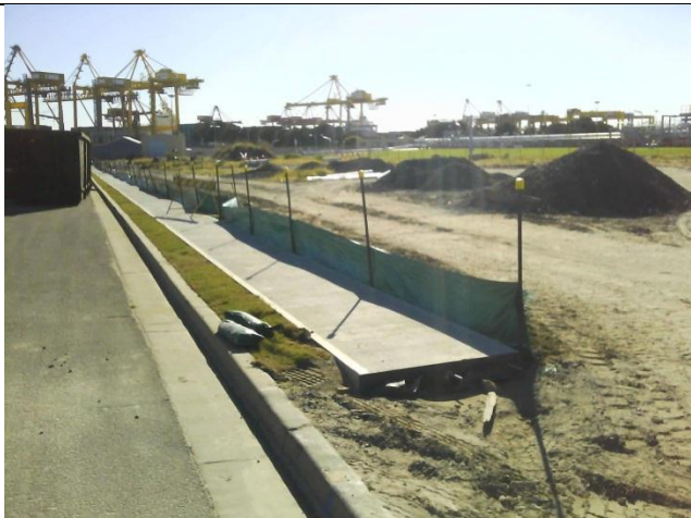
Photo 11 Sediment controls in place in vicinity of small stockpiles
