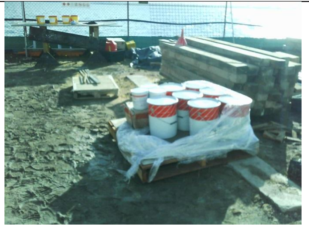
Photo 21 Further drums of Class 9 substance stored without secondary containment.
