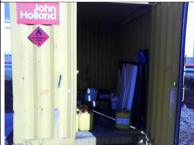
Photo 14 Bundled, ventilated storage container for hazardous substances
