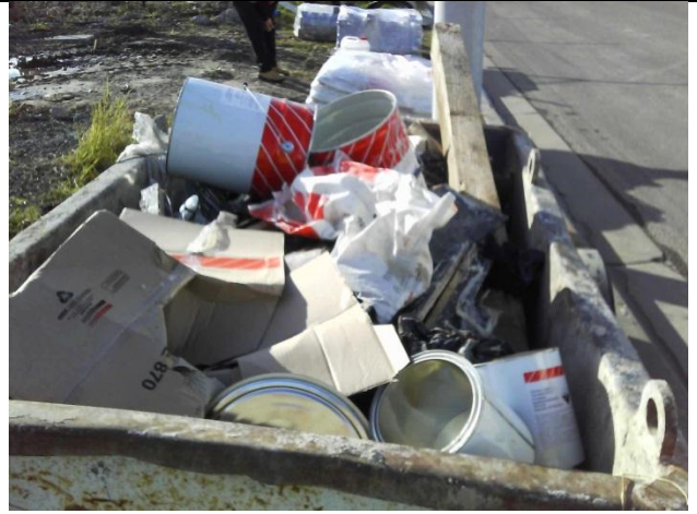
Photo 27 Empty drums with residues within the general waste skip
