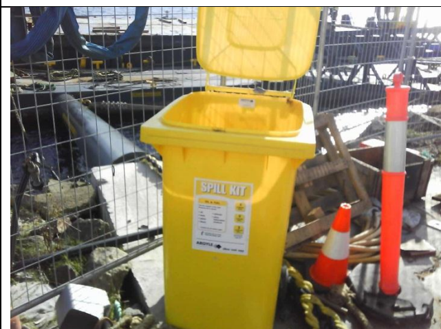
Photo 16 Spill kit near the foreshore – contents depleted
