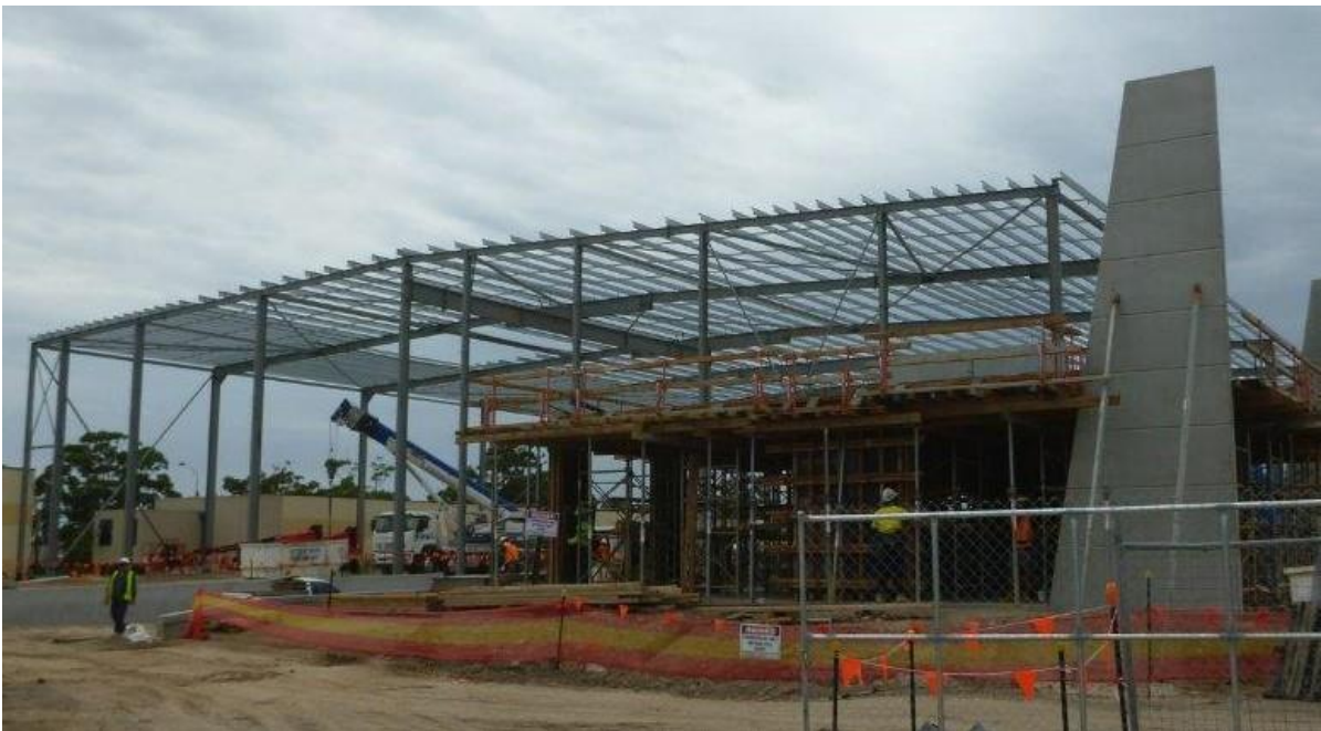
Construction of Warehouses – Precincts C and F
