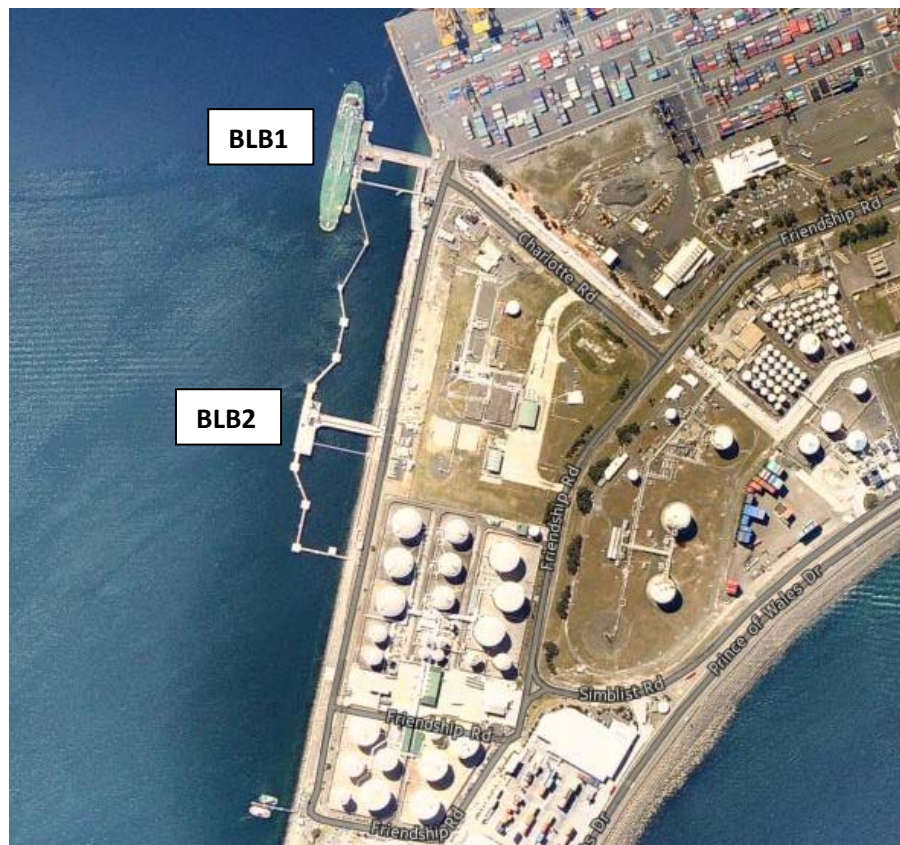
Figure 1: Location of BLB2 infrastructure
