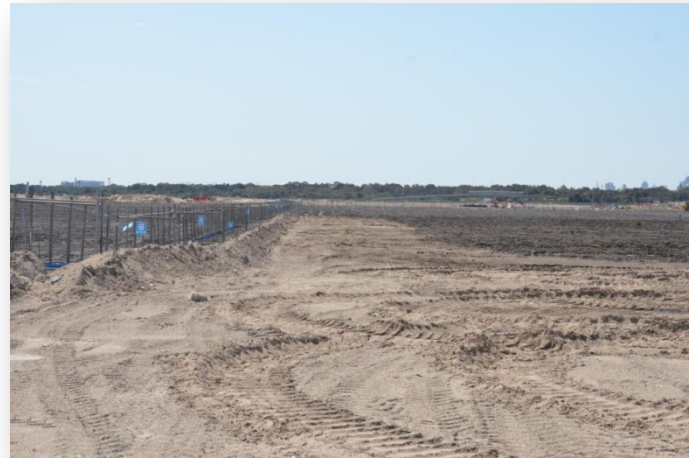
Silt fence and bunding
