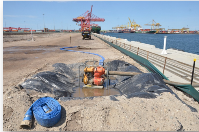
Silt fence and bunding
