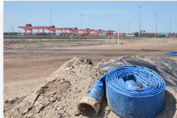
Knuckle as at Oct'12 (Looking west towards existing terminal)
