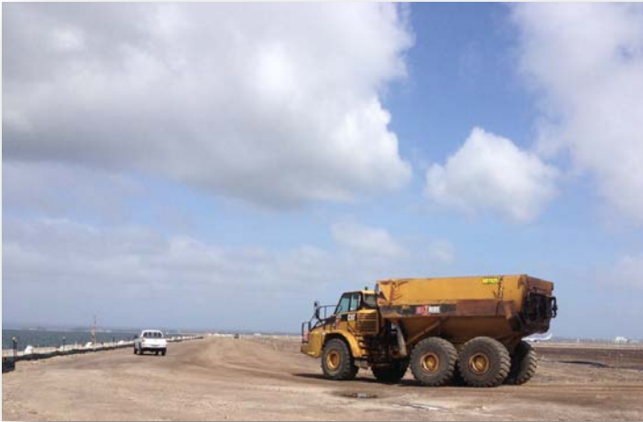
Applying Dustbloc to the Knuckle
