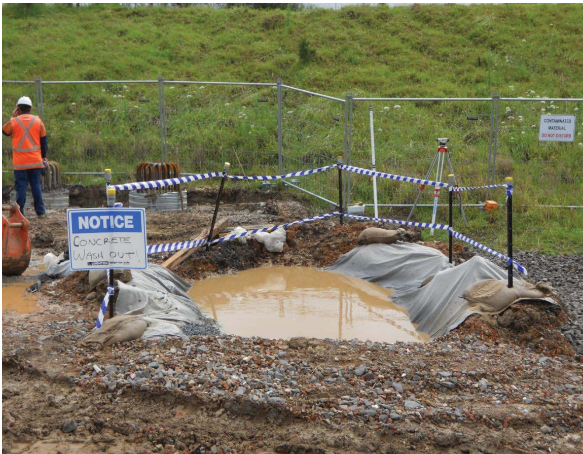
Plate 1: Good practice concrete washout controls associated with road over-bridge works
