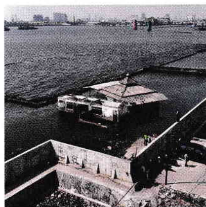
A giant sea wall in Jakarta, Indonesia, will protect the city
