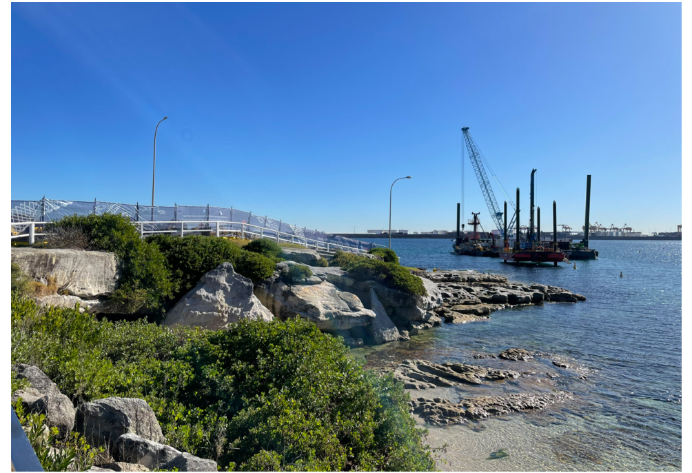
Piling crane barge La Perouse
