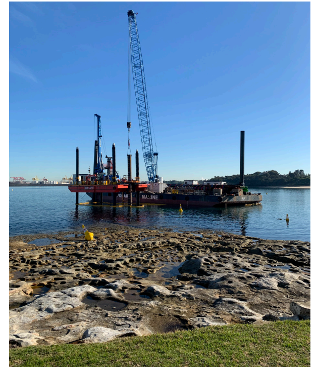
Piling, La Perouse
