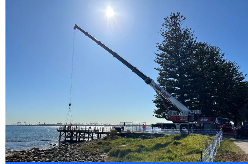
Removal of viewing platform, Kurnell
