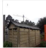
2. Precast Concrete Hut 1
