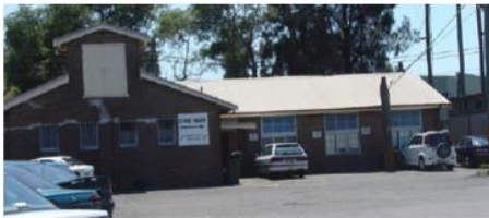
1. MCS HRT Admin Building
