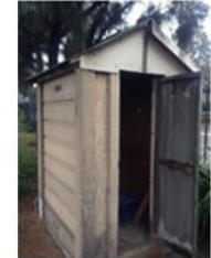
3. Precast Concrete Hut 2
