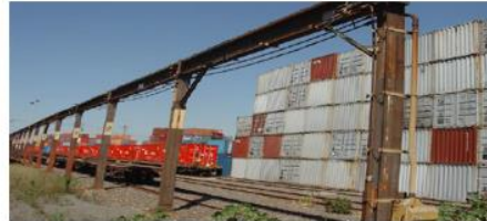
5. The Electric Overhead Travelling Crane
