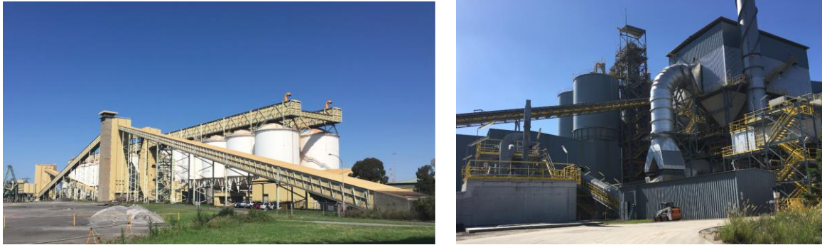
Figure 15. Examples of the use of consistent design solution to integrate buildings, silos and covered areas
