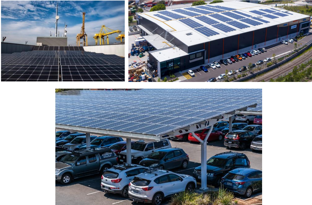
Figure 3. Examples of rooftop and shade structure onsite solar applications
