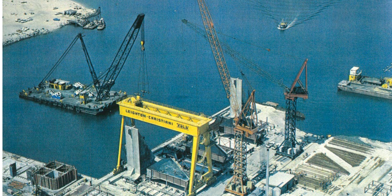
Counterfort wall unit pre-cast yard (1978)
