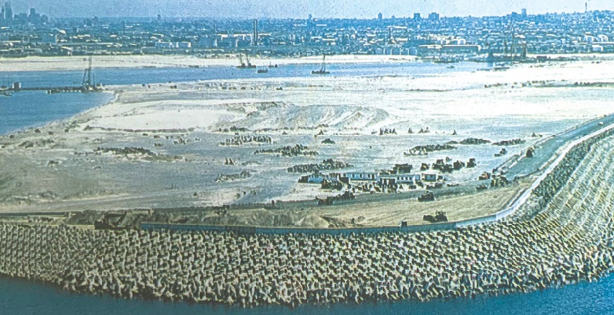
Construction around the Port Botany revetment wall (1978)
