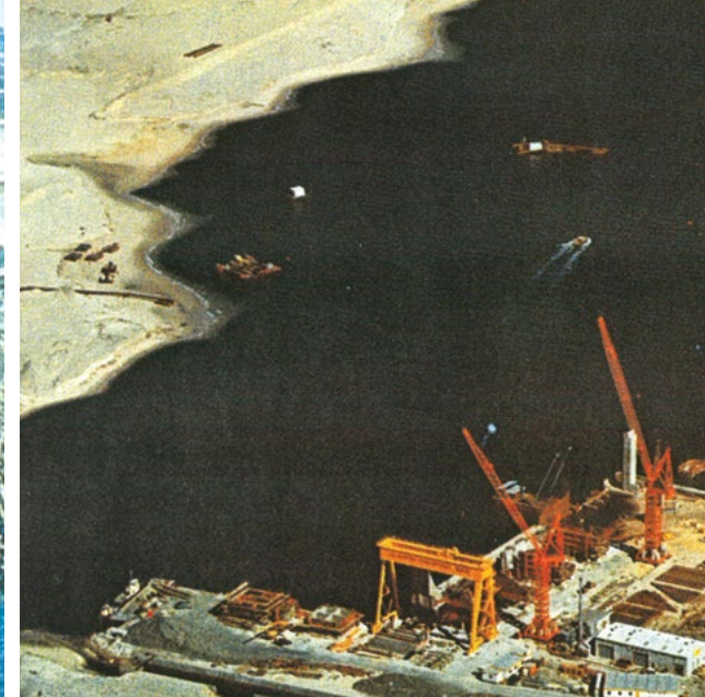
Brotherson Dock construction (1978)
