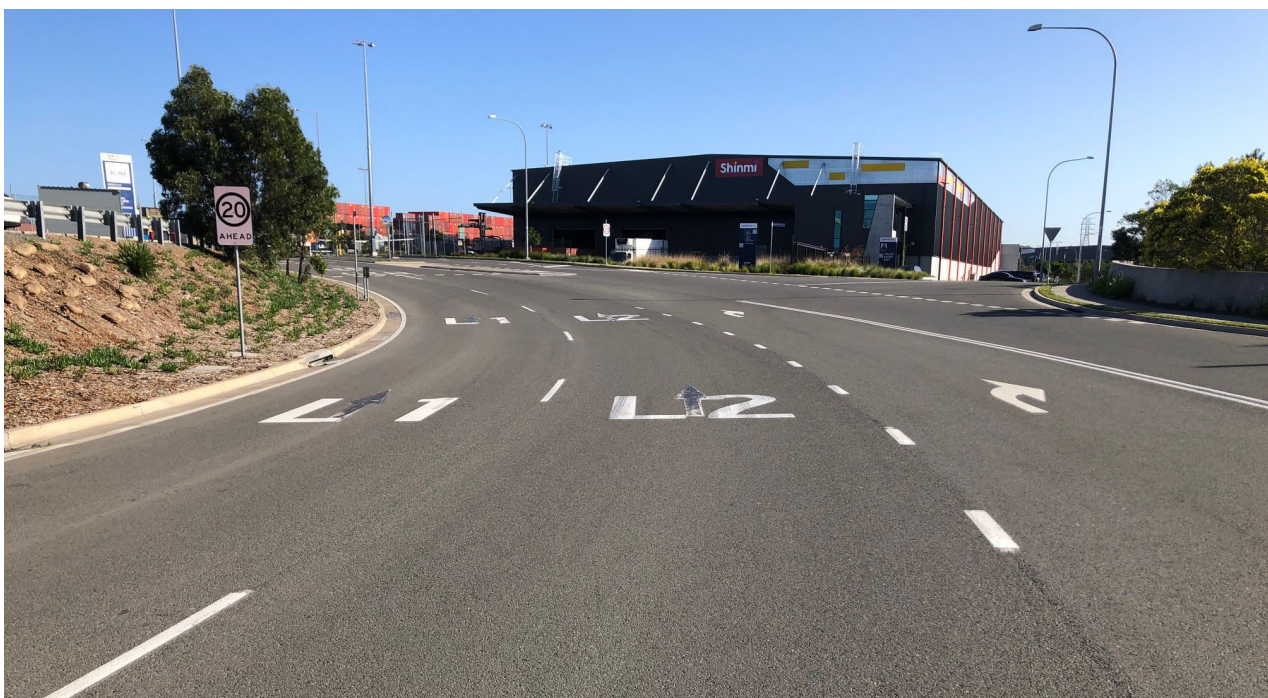
Figure 3: Example of Linemarking and Directional Arrows on Site
