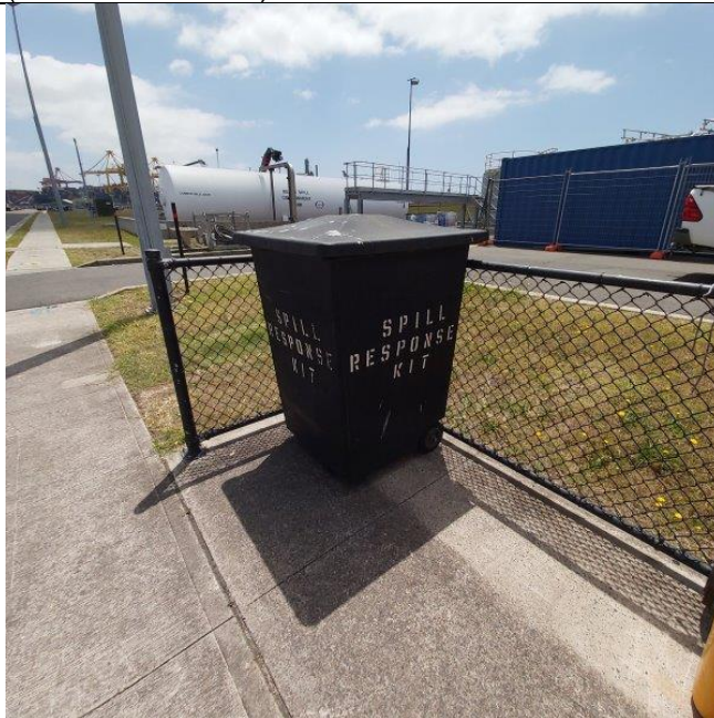
Backup spill response kit near BLB2 Operations centre (spill kits also supplied by users during transfer operations)
