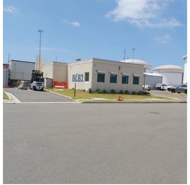
View of BLB2 operations centre / office
