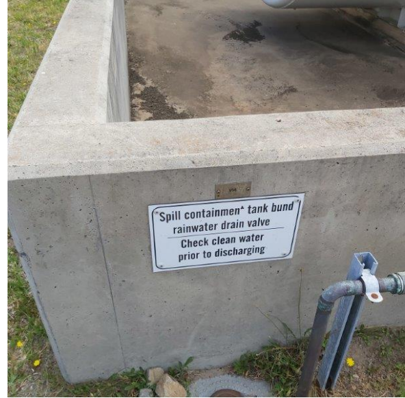
Signage on the spill containment tank
