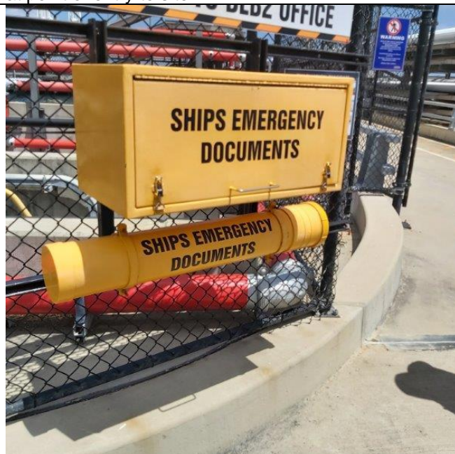
Ships Emergency documents stored in the box or tube during transfer operations (had not yet been transferred – set up in progress at time of audit)
