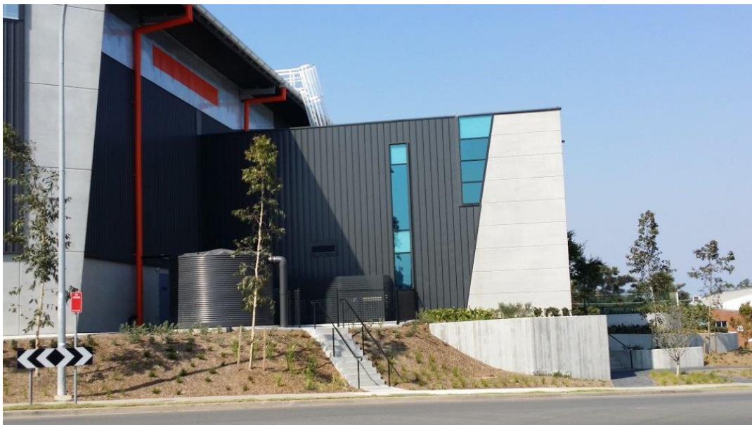
Warehouse C1 rear - landscaping and rainwater harvesting surge tank
