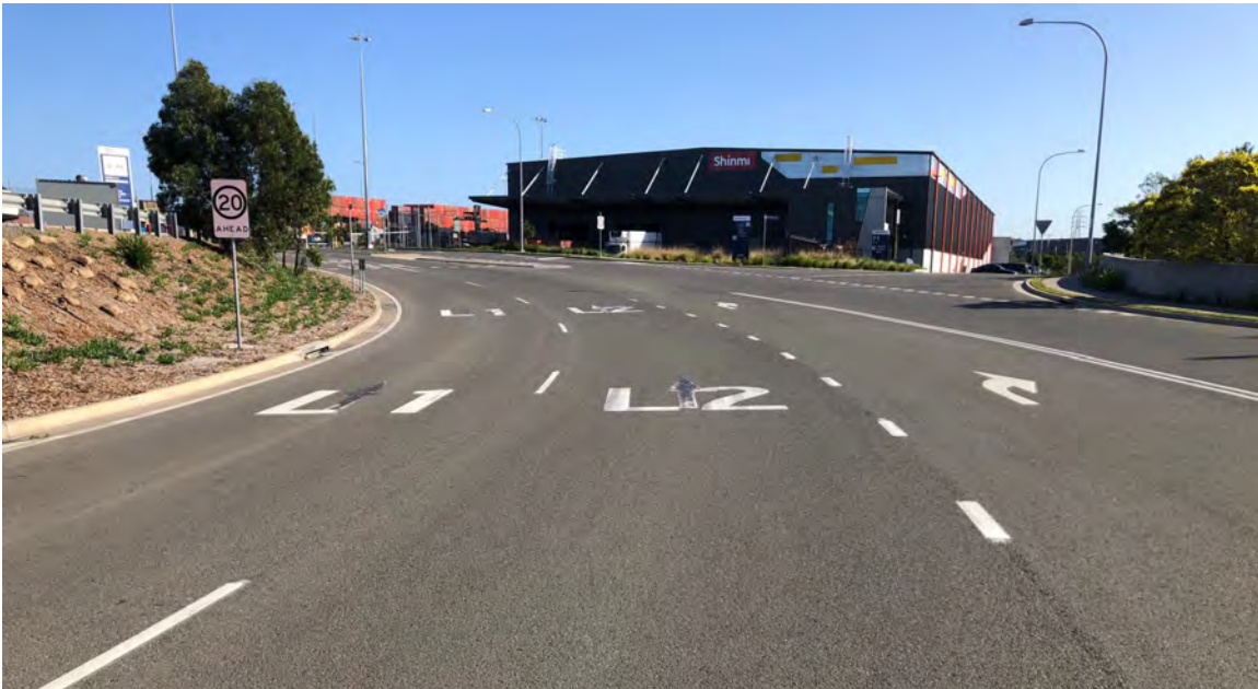
Figure 2: Example of Linemarking and Directional Arrows on Site
