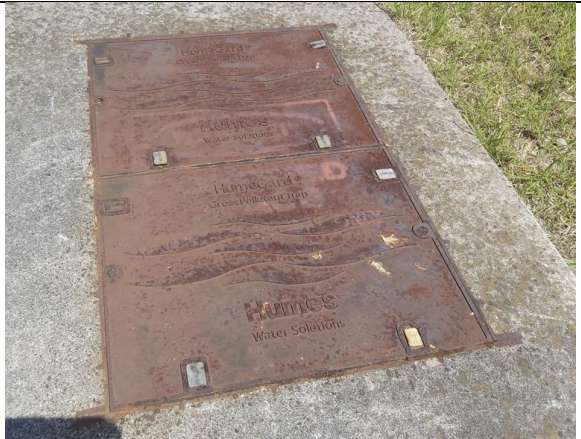
Humes Gross pollutant trap /oil water separator (underground). Cleaned out annually
