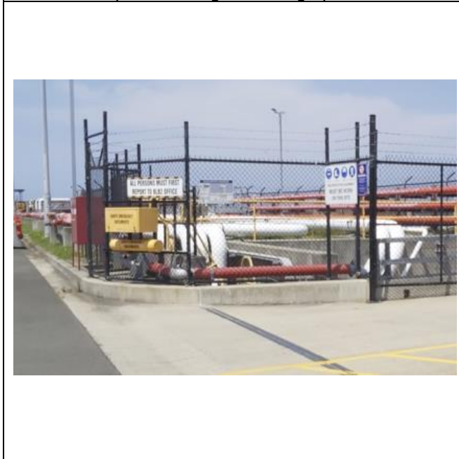
Emergency document box and tube for current documents relating to products being transferred
