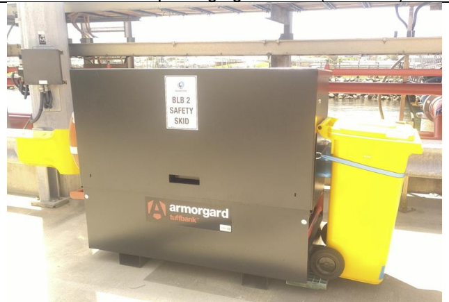
Quantem BLB2 Safety skid – includes spill kit and personal protective equipment for emergency use
