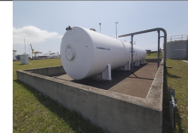
Berth spill containment tank (empty) – fully bunded. For use in case of spill at the berth and on site
