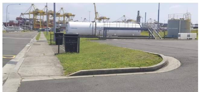
Berth spill containment tank (empty) – fully bunded. For use in case of spill at the berth and on site
